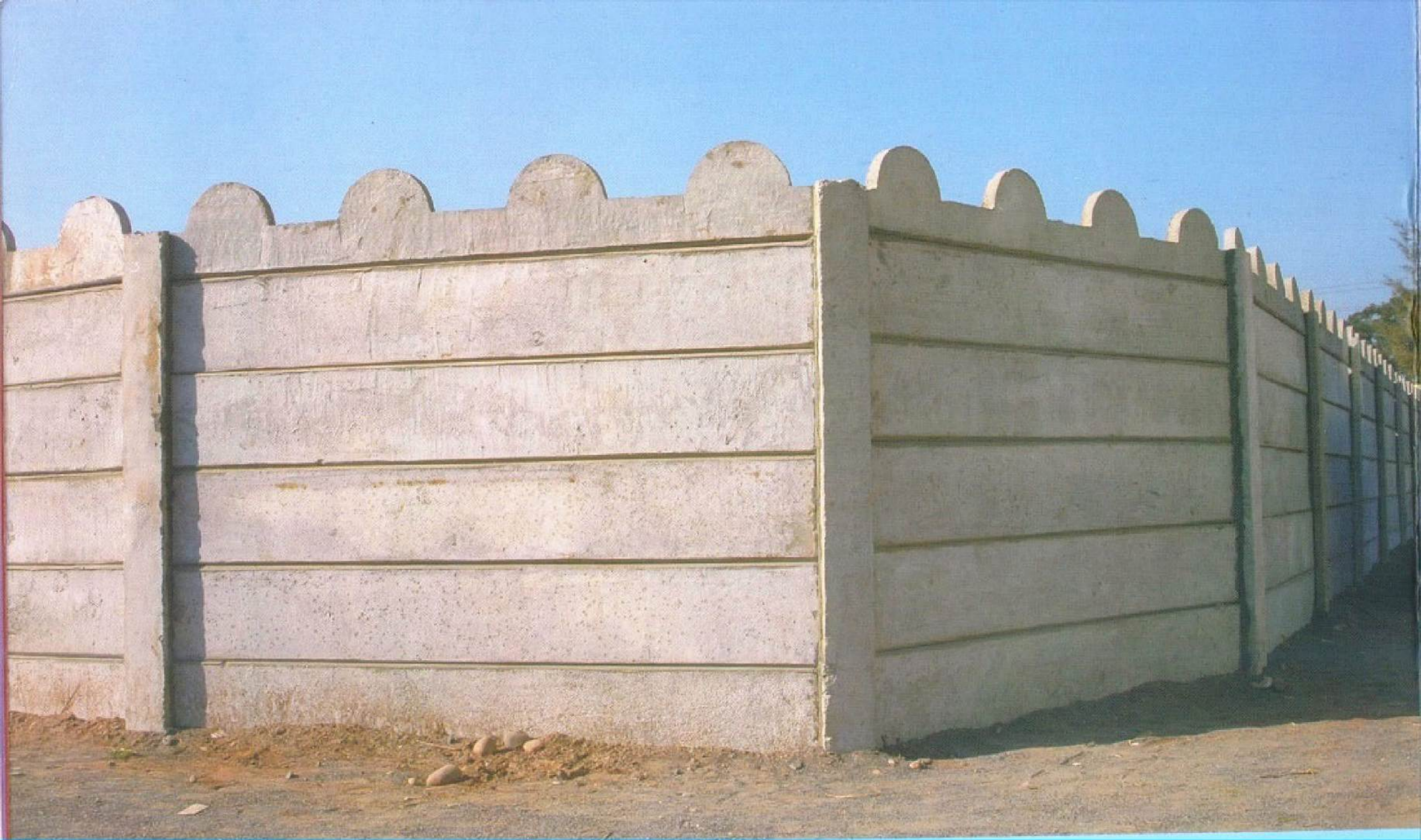
Final Finished Compound Wall
