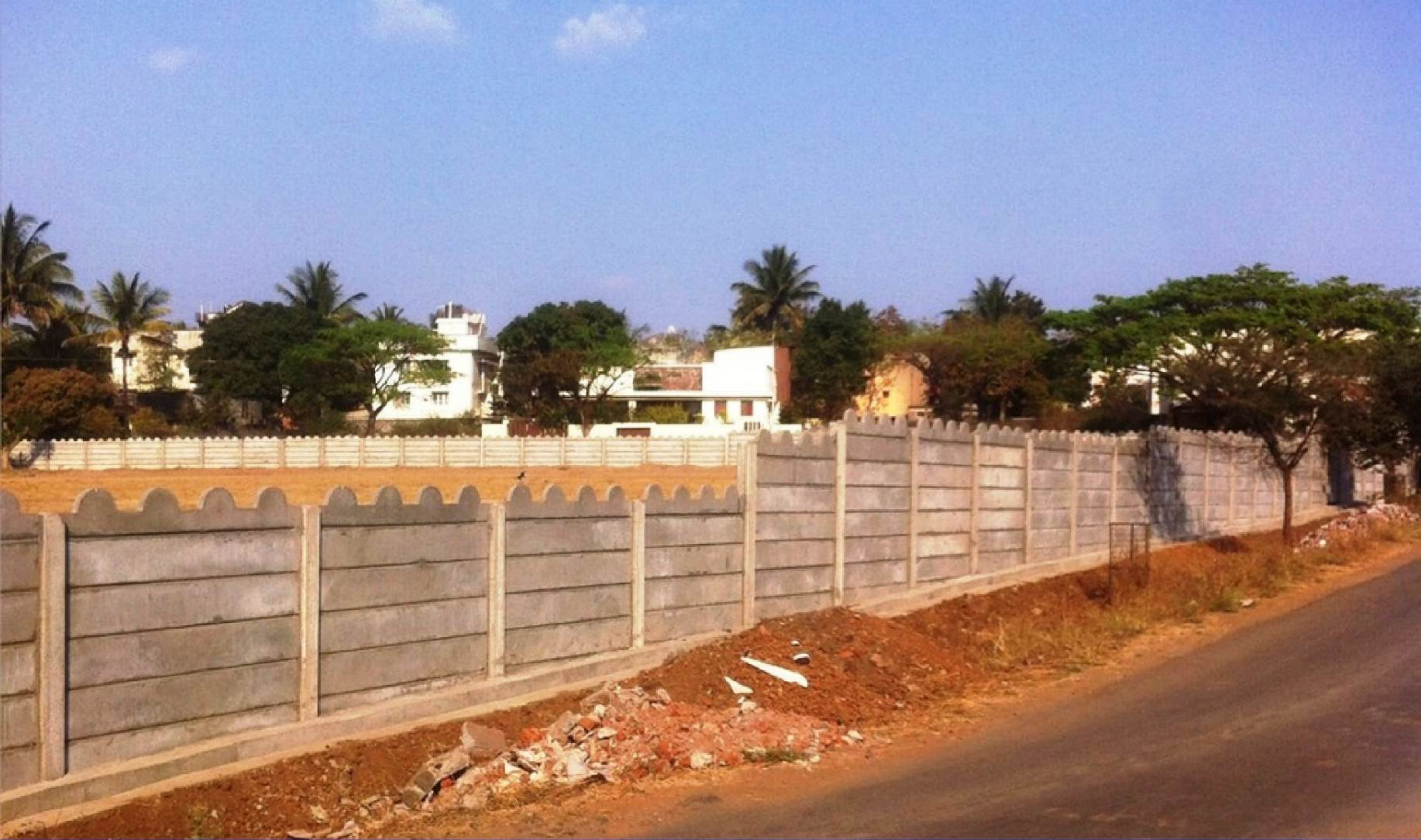
Housing Society Compound Wall
